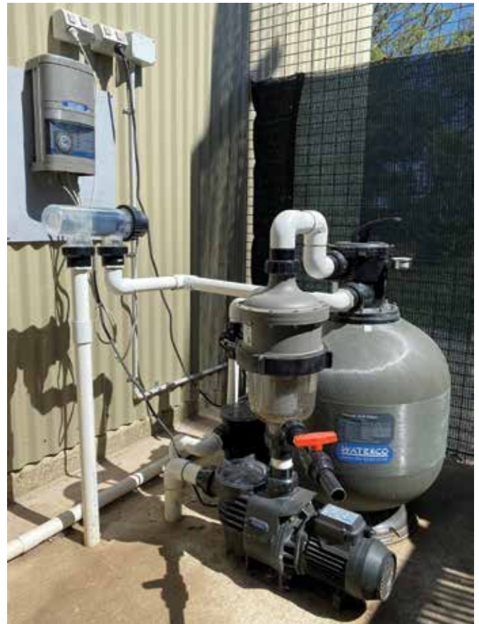
Specialising as a first-stage filter, MultiCyclone stops up to 80 per cent of the incoming dirt load, easing the workload of the pool's filter media.
