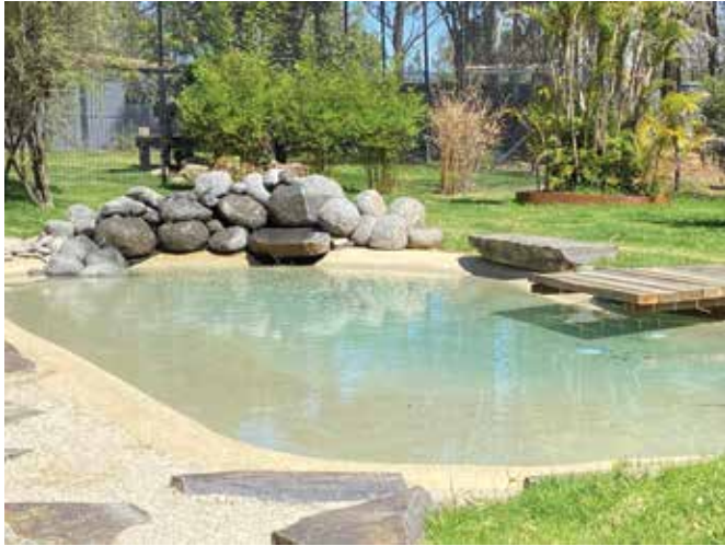
The tiger pools are continually crystal clear, and backwashing is at a minimum with the use of Waterco's MultiCyclone.
